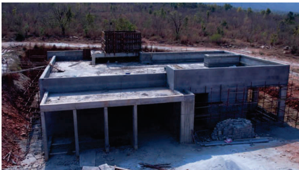
Sports Utility Block construction
