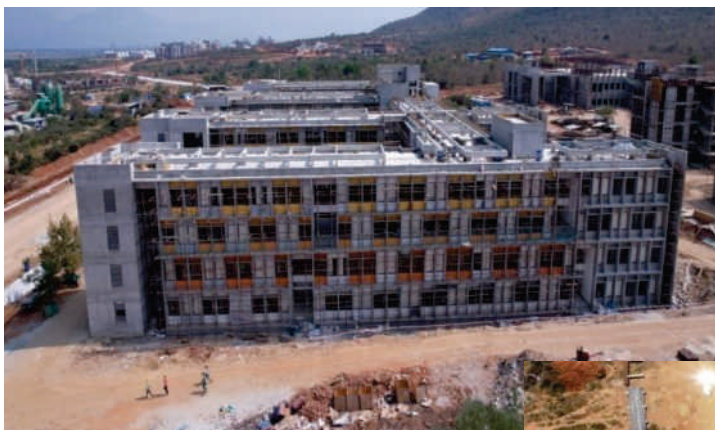
Hostel Block-1 construction
