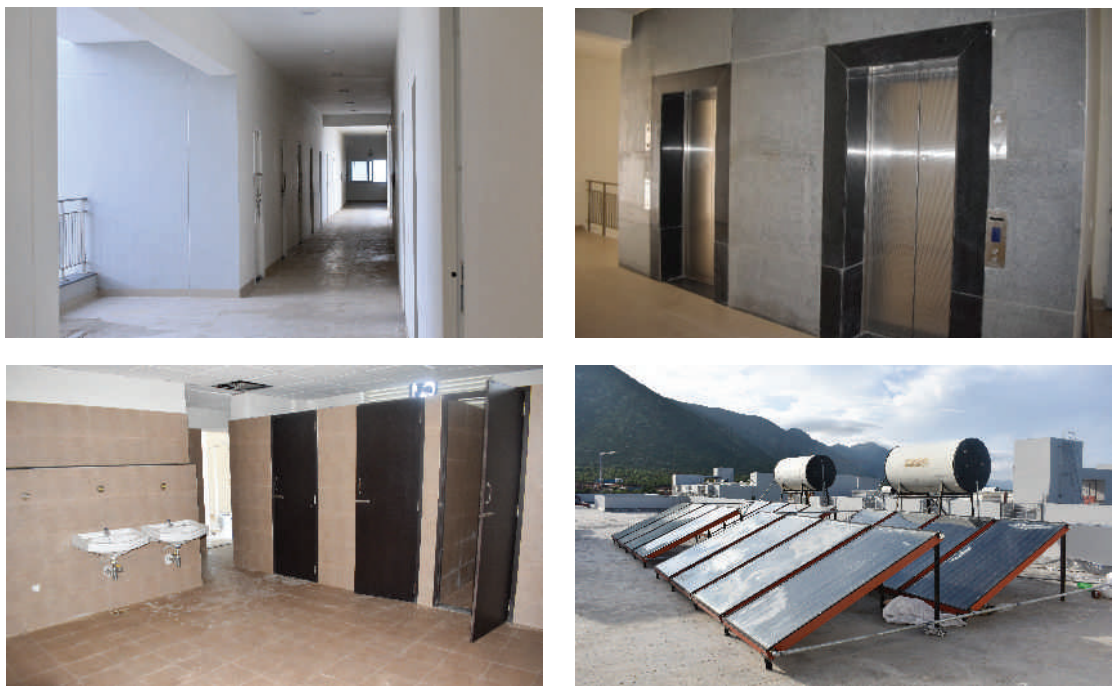
An inside view of the Hostel Block – F
