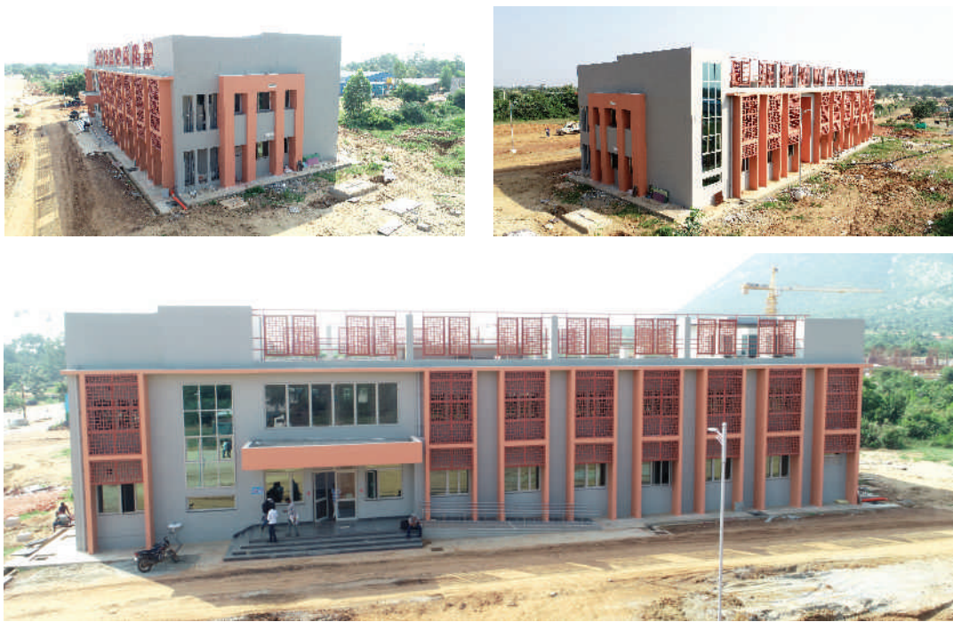
Outside view of the Engineering Unit Building
