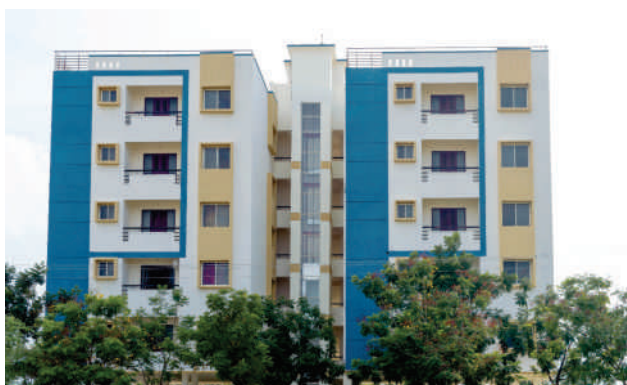
Guest House facility at KCR Towers
