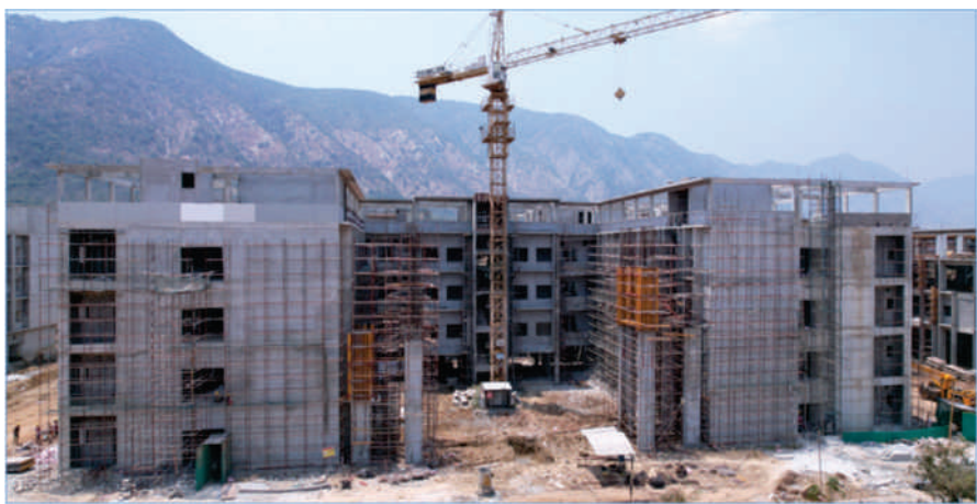
Department Block-1 construction
