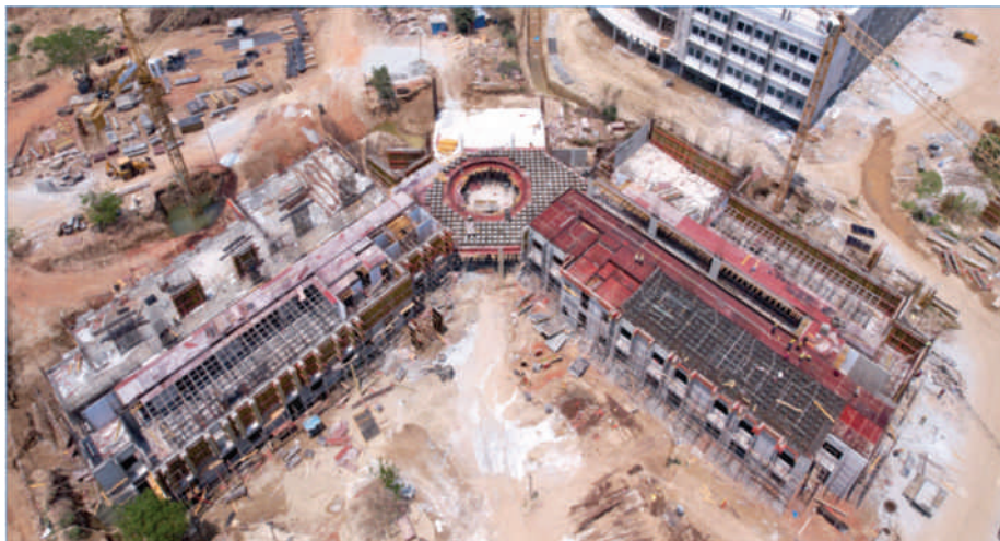
Lecture Hall complex construction
