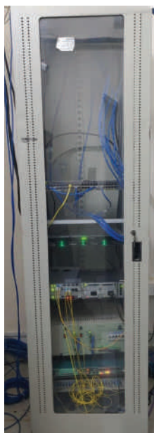
Sophos-330 XG firewall and network rack
