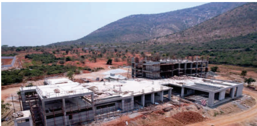
Visitors Hostel Construction
