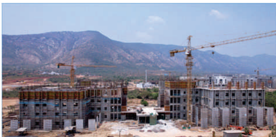
Administrative block construction
