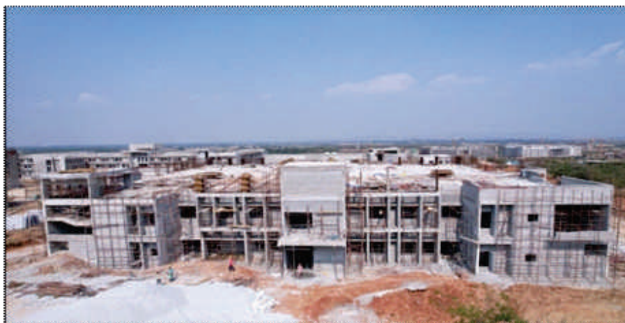
Dining Block construction
