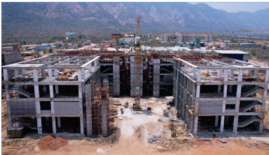
Central Instrumentation Facility Building construction
