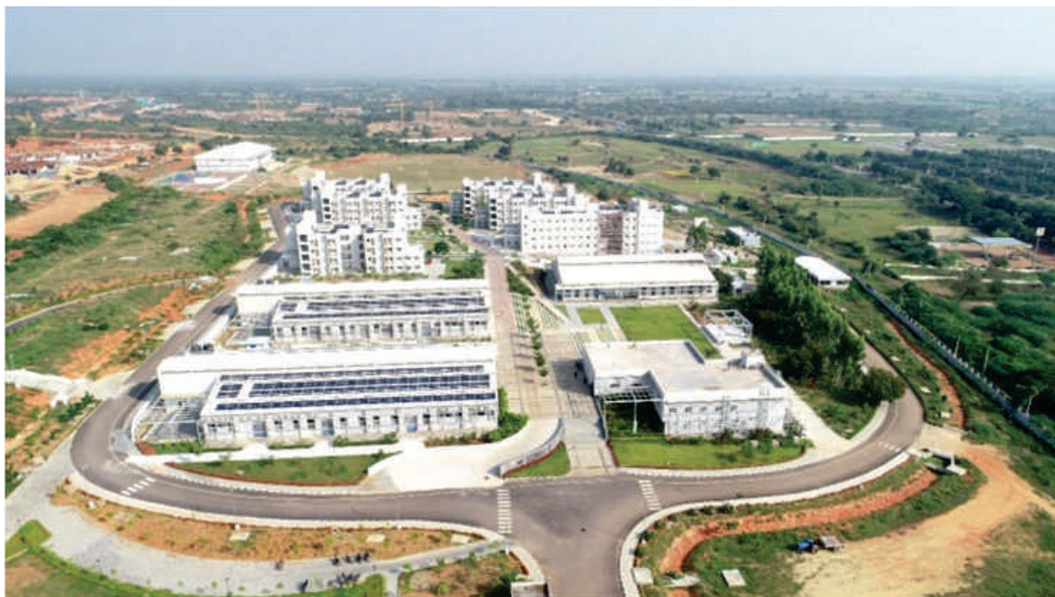
An aerial view of Phase -1, Stage 1A of the permanent campus
