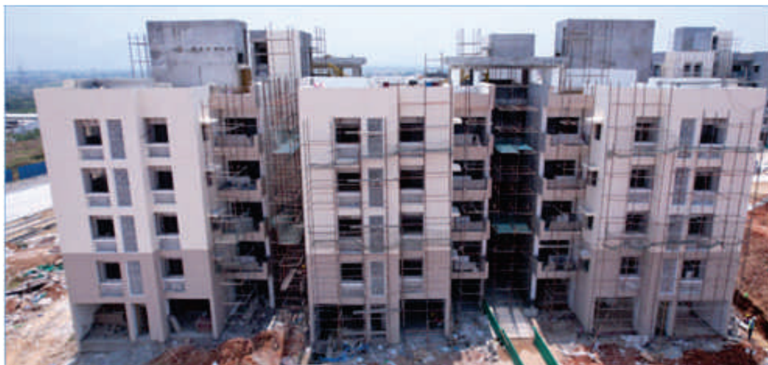
Type-D Block construction
