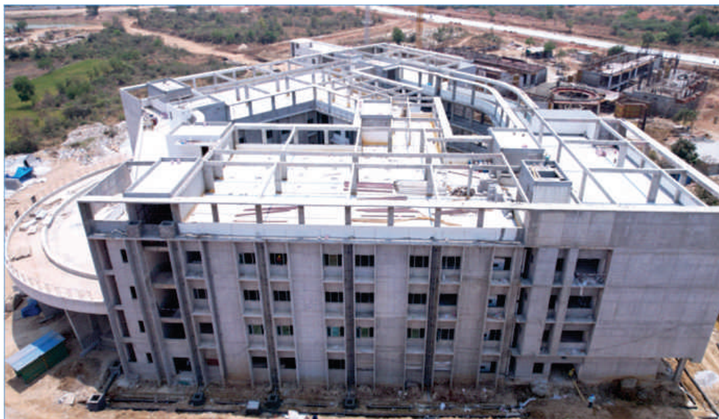
Department Block-2 construction
