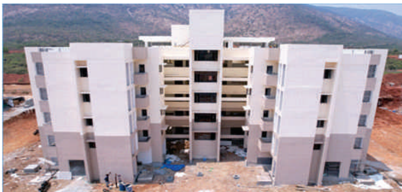
Type-C3 block construction
